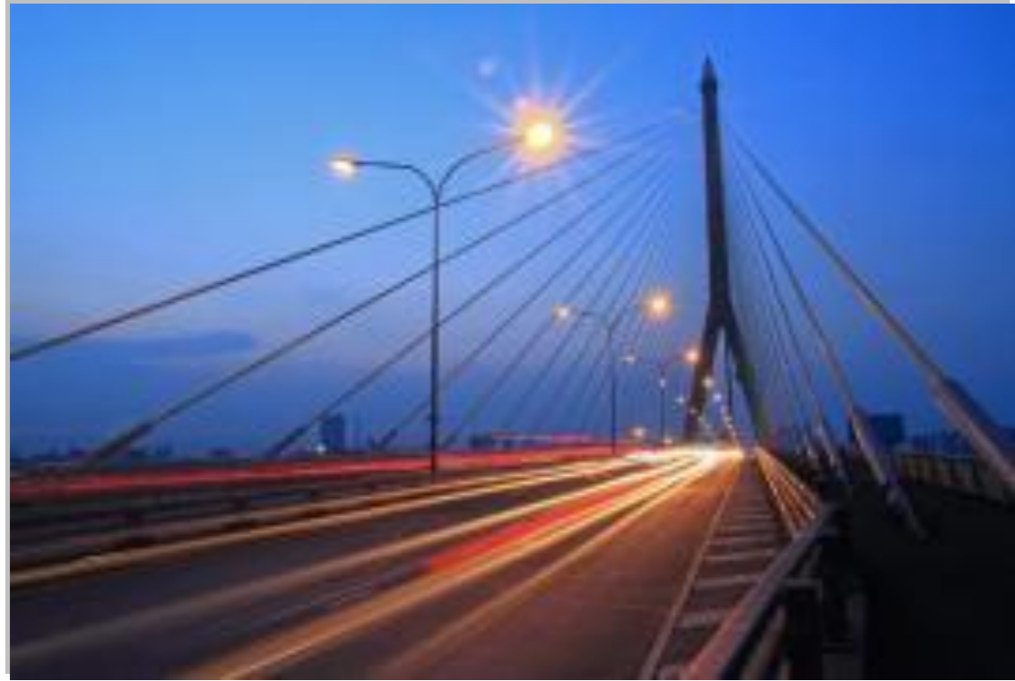
Lighting & Distribution Poles
