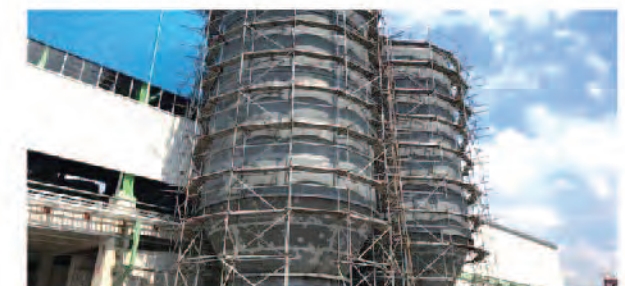
不锈钢304+Q345R- CLC越南造纸厂纸浆塔 Supplied SS Clad Plates 304+Q345R to CLC for Vietnam Paper Mill
