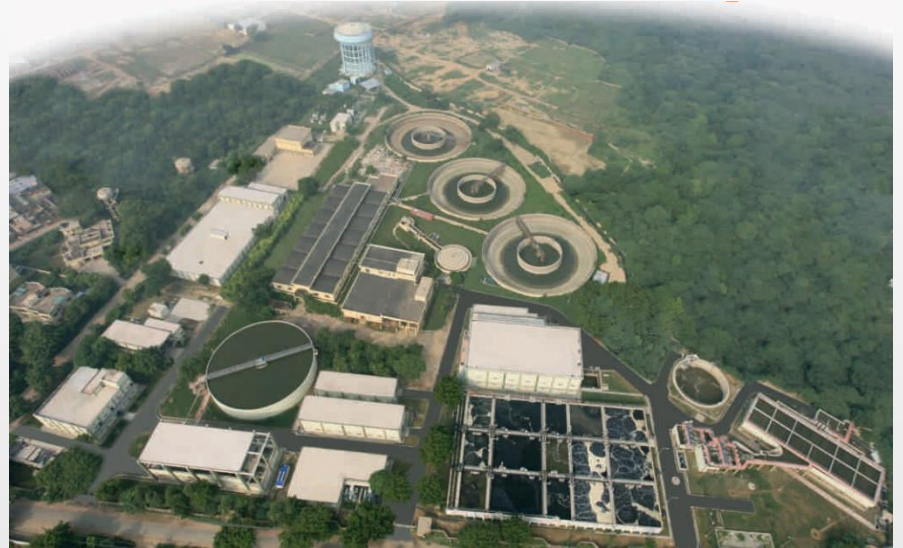
Drinking Water Treatment Plant - Agra, India
